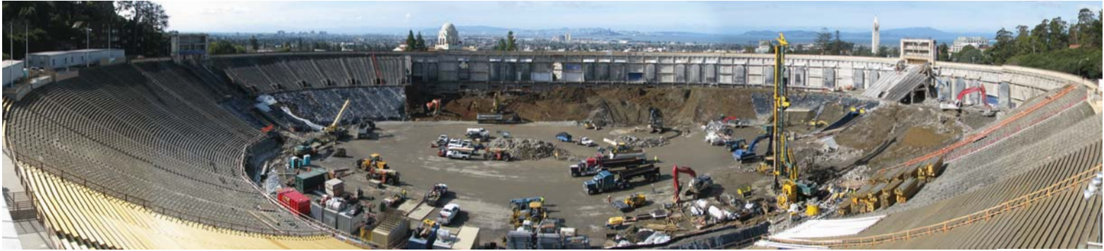
California Memorial Stadium, CA
